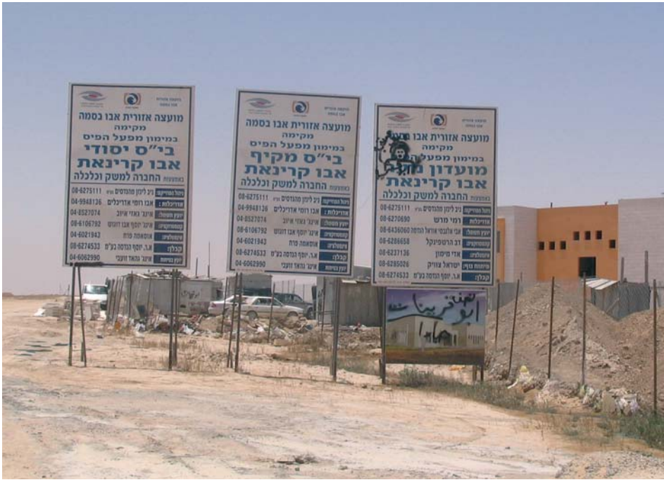
Figure 2: Construction of educational and public institutions in the village of Abu Krinat in the Abu Basma Regional Council
