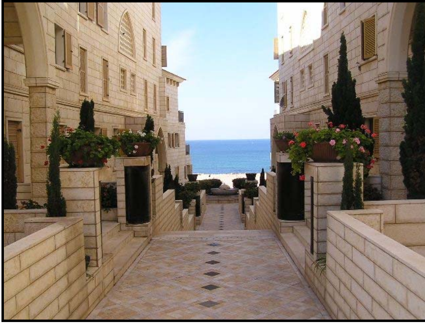
Photograph: The Andromeda Hill project. For further photographs, see the HRA website: http://www.arabhra.org/Hra/ImageGalleries/ImageGalleryPage.aspx?ImageGallery=6752&Language=2
