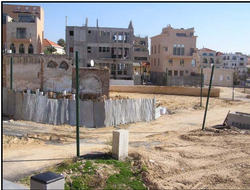
Photograph: Urban neglect in the Ajami neighborhood
