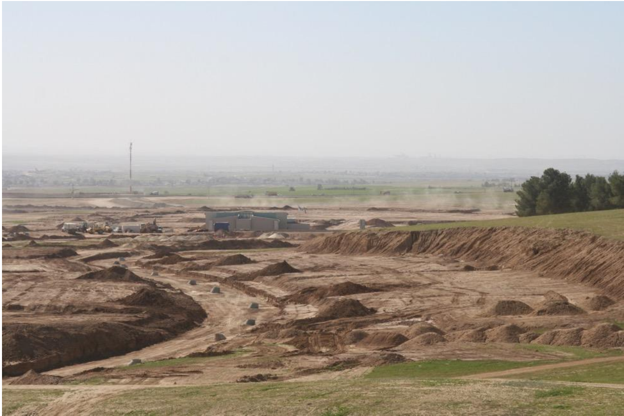
Construction of Karmit's sewage system. Photo: Michal Rotem.
